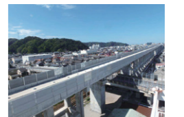
No. 3 South Fukui Viaduct
