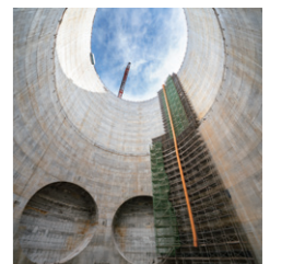
Linear Chūō Shinkansen Kajigaya emergency exit and materials delivery entrance
