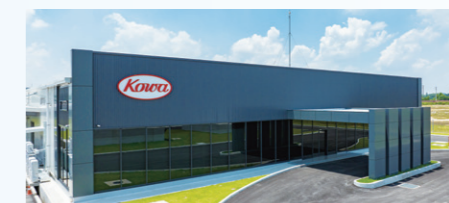
Kowa General Foods (Vietnam) Co., Ltd. Factory Project
