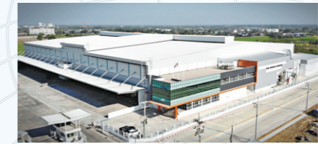
All New Complex Phase 2 Project
